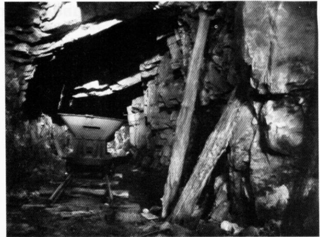
Reconstructed track and tipping wagon in the uncompleted section of the Jersey War Tunnels (Ho8) . Photo Adrian Armishaw
